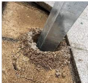
Stolpe sat i beton
